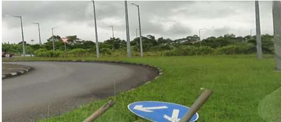
Figure 41: Broken Traffic Sign at Flacq
