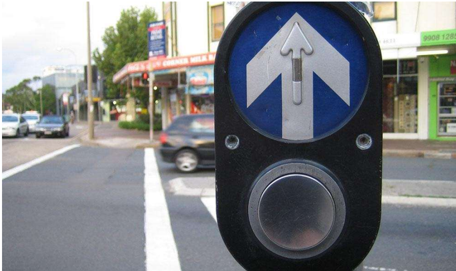
Figure 39: PB/5 press button Australian design to assist vision and sound impaired persons
